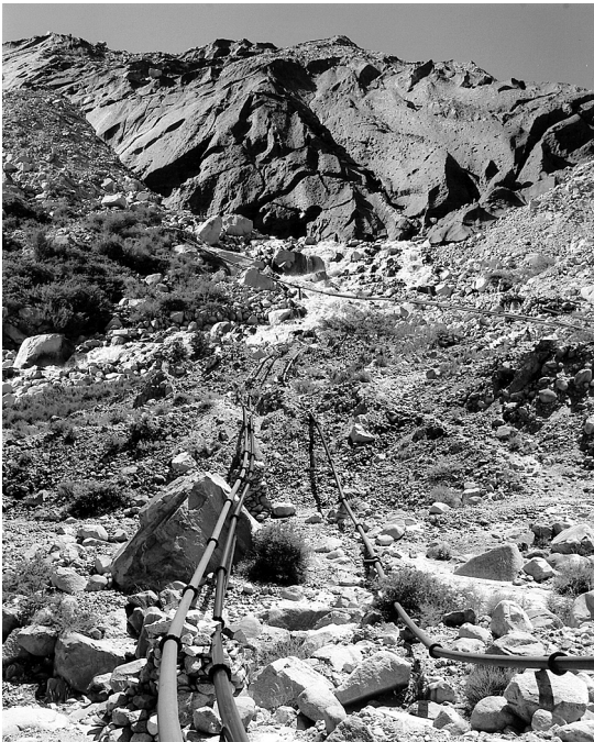
Photo 4. Irrigation from the Gulkin glacier using steel pipes (Photo: 31 August 2007).
